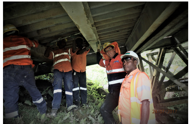
Bridge repair, PNG
