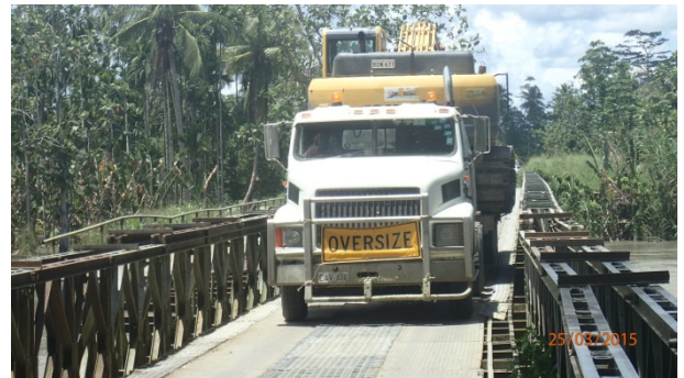
Trafficability Load Limit assessment, Angabanga Bridge, PNG
