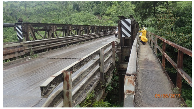
Bridge assessment and repair, PNG
