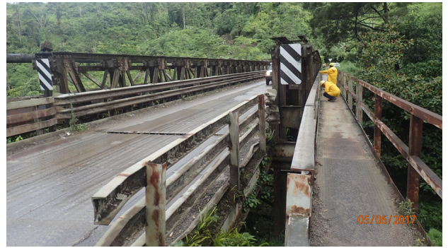
Bridge assessment and repair, PNG
