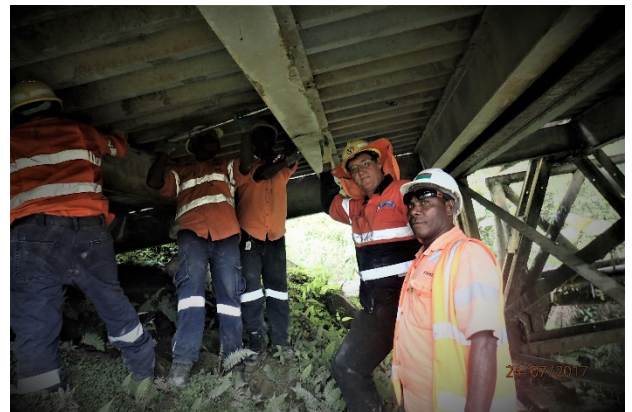
Bridge repair, PNG
