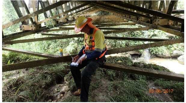
Bridge inspection & condition assessment, PNG
