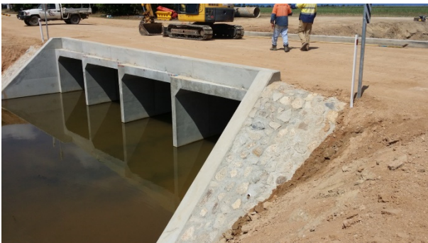
Flood damaged culvert replacement, North Queensland
