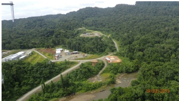
Gas well construction camp, Gulf Province, PNG
