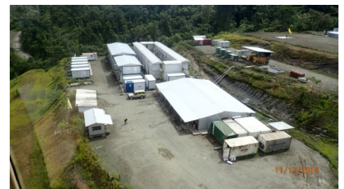
Rig site construction camp, Gulf Province, PNG
