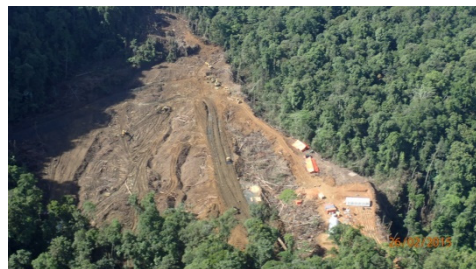
Construction of Gas well camp, Gulf Province, PNG
