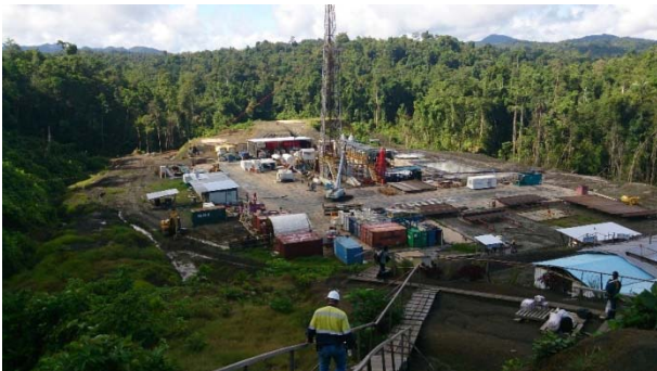
Infrastructure at drill rig site, Gulf Province, PNG
