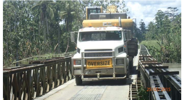
Trafficability Load Limit assessment, Angabanga Bridge, PNG
