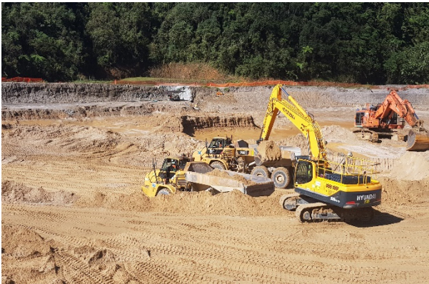
Construction of dam, PNG
