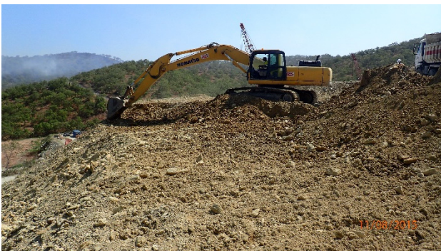
Bulk earthworks project, PNG
