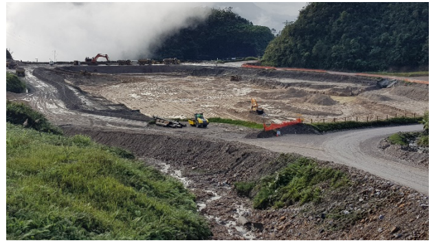
Dam Construction, PNG
