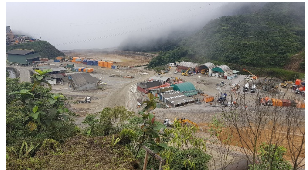
Infrastructure Construction, PNG
