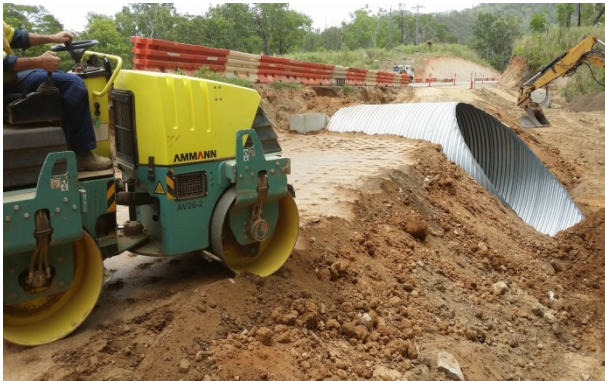
Highway reconstruction, North Queensland
